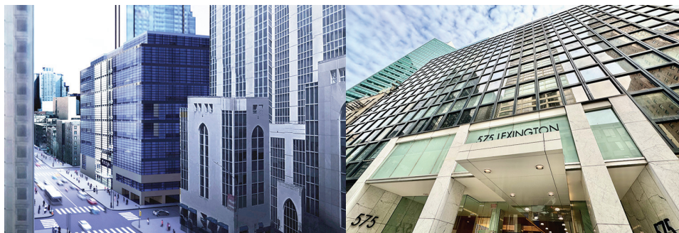
Exteriors of 1334 York Avenue, left, and the Midtown Clinical Care Center at 575 Lexington Avenue, right.
